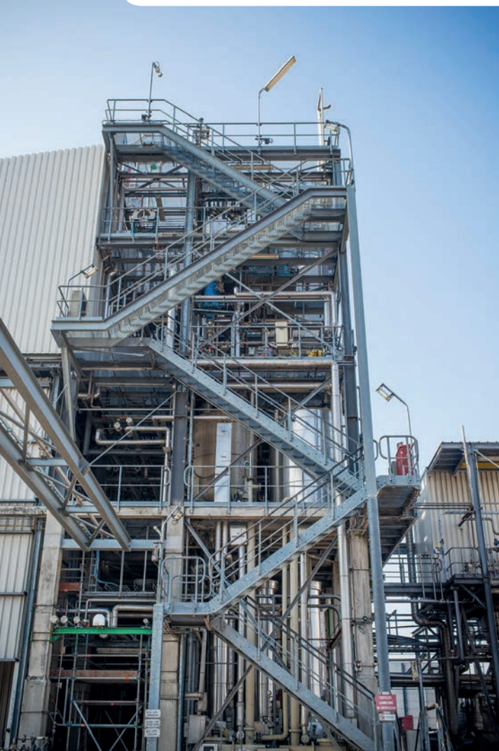
Proviron's current binder plant in Ostend
